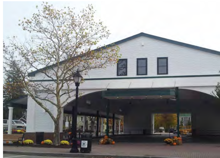
The Waterhouse Center in Kennebunk, Maine is an open-sided pavilion that hosts ice-skating in winter and pickleball courts in summer. Photo credit: Waterhouse Center Facebook Page.
