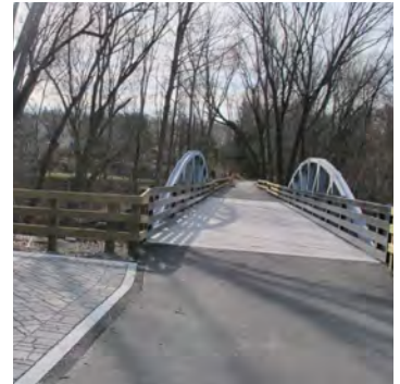
Bruce Freeman Rail Trail (2019 and ongoing)
